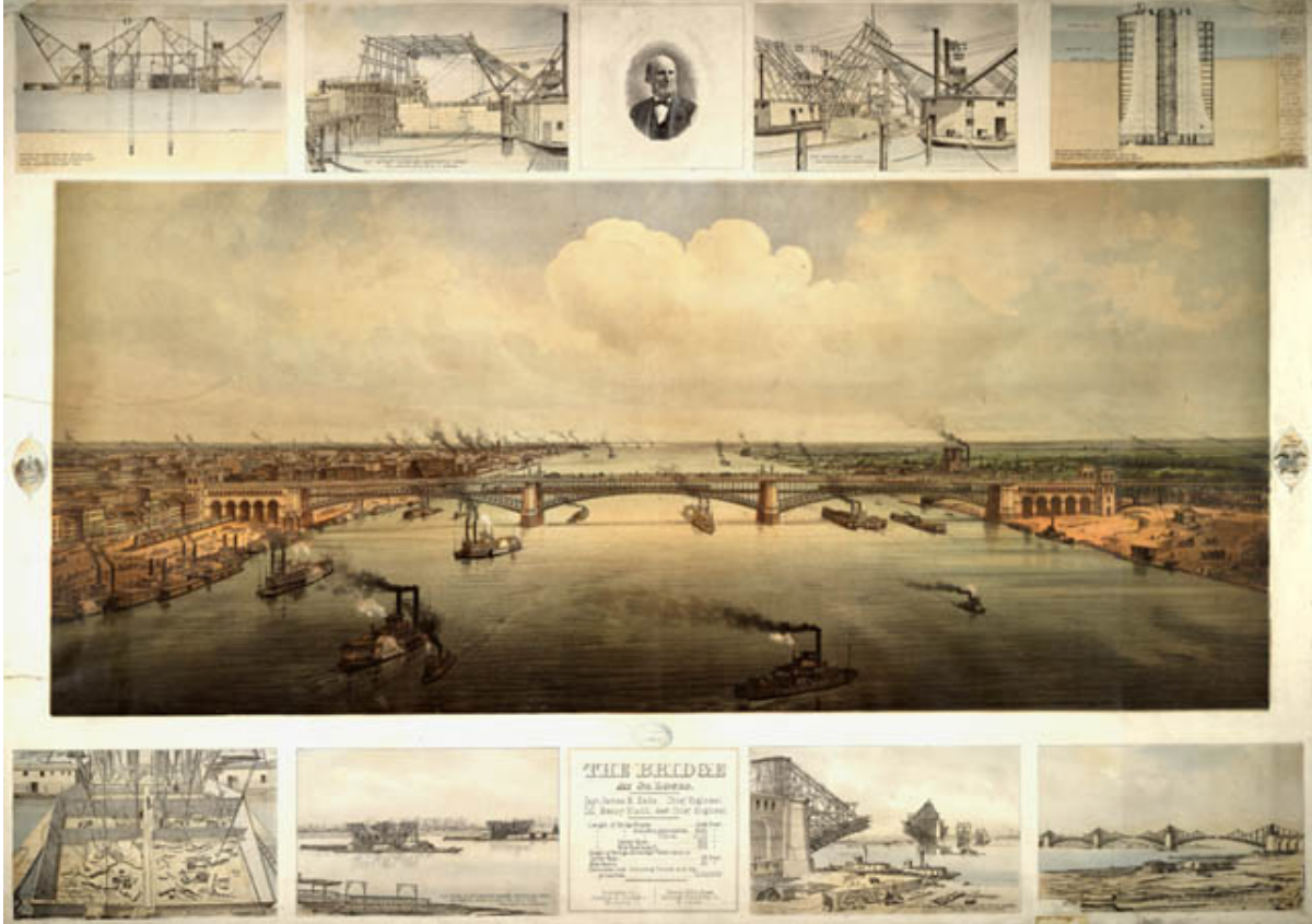
Eads Bridge over the Mississippi River, St.Louis, MO
